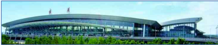
WUHAN TIANHE INTERNATIONAL AIRPORT
